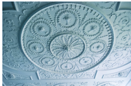
Decorative plaster ceiling at Kenmore. ("Fredericksburg, VA - Kenmore Plantation 03.jpg" by Jrozgado is licensed under CC BY 4.0)
